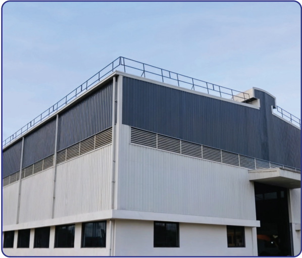
Location : Padra, Gujarat, India
